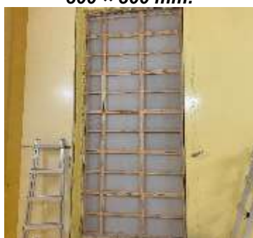
b. The frame spacing was set at 600 × 300 mm.
