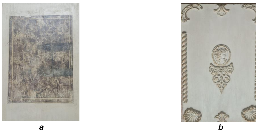
Fig. 25. a-Finish made by transfer technique, b-Finish with moulded ornaments.
