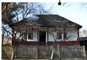
south facade entrance porch - sala
