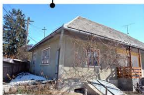
facade facing the street
