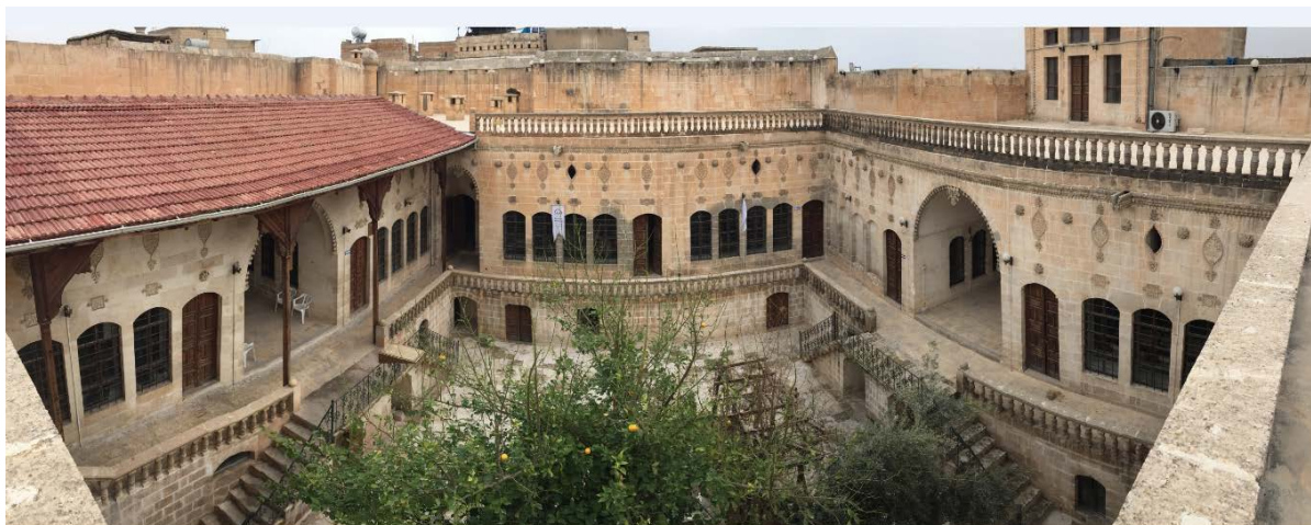
Fig. 1. The blocks of the building at the wings of the courtyard (Author).
