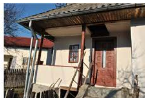
detail of wooden railing - facade
