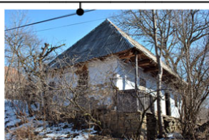
view of the main facade
