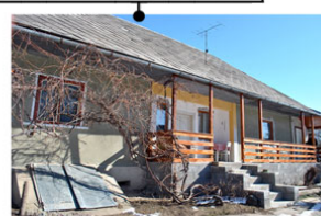
view of the south facade
