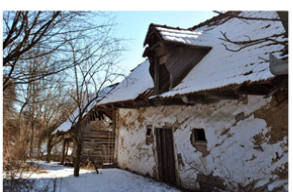
view of the annexes
