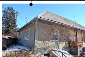
south facade facing the yard
