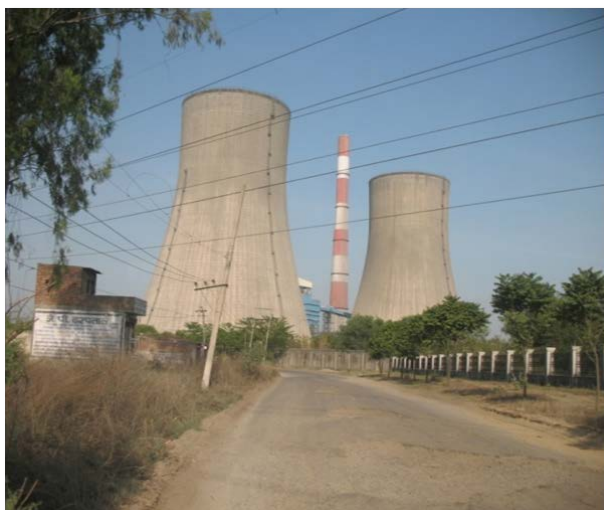
Fig. 2. Cooling tower in Thermal Power Station.
