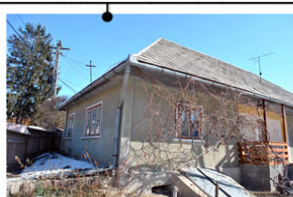
facade facing the street
