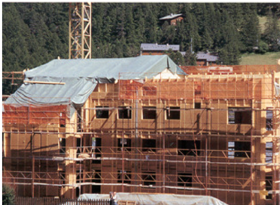
b – Montajul unei case multietajate din plăci stratificate din lemn masiv / Assembly of a multi-storey house made of laminated solid wood panels. Foto: Nägeli Holzbau AG, Switzerland
