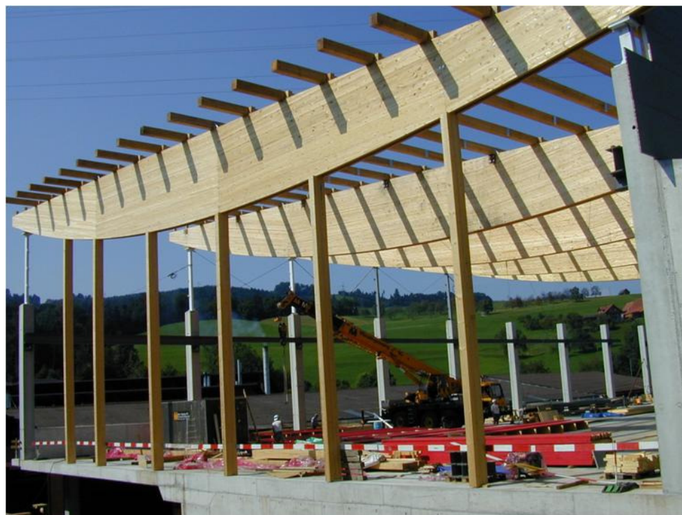
c – Plăci stratificate din lemn masiv folosite ca elemente constructive supuse la încovoiere / Solid wood laminated panels used as structural elements subjected to bending. Photo: Schilliger AG, Switzerland
